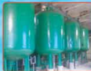
Iron Removal Plant
