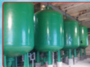
Iron Removal Plant
