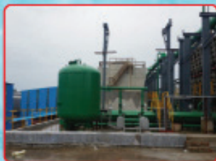
Filtration for Cooling Tower Make up
