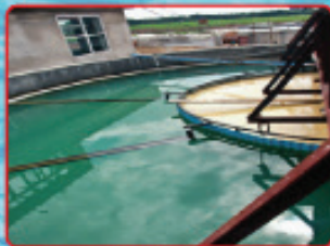
High Rate Solids Contact Clarifier
