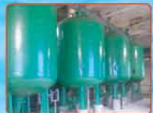
Iron Removal Plant
